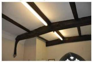
The lighting makes up a relatively small overall energy load within the building. The church has clearly made a dedicated effort to up-grade the majority of the lamps in the church over time to LED fittings. There are however a small number of lamps which are still the relatively inefficient fluorescent and SON fittings.
