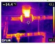
The pipework within the plant room has the majority of its straight lengths insulated but the more complex shaped pipework fittings, such as valves, have been left uninsulated. These exposed areas of pipework contribute significantly to wasted heat loss from the system and make the plant room unnecessarily warm. The exposed hot surfaces also represent a health and safety risk of burns for those working in the area.
